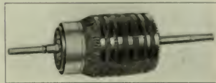
FIG. 4. A COMPLETE ARMATURE
